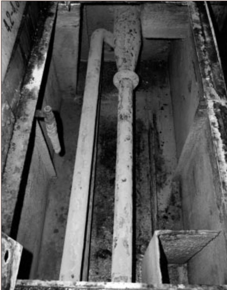
Fig 8 Encrusted temperature sensor
